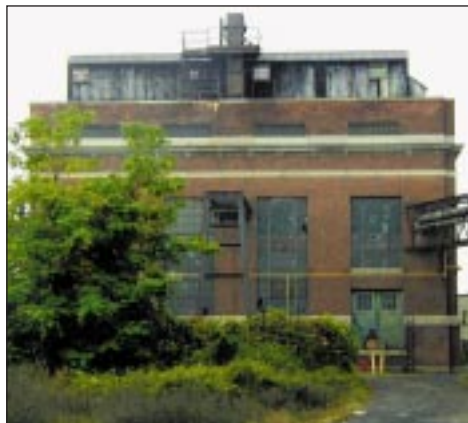
52 space heaters provide heat for tenants at the Springfield Industrial Center.
