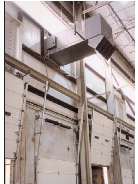
Direct Gas-Fired Space Heater High Efficiency, Blow-Thru Design Source: Cambridge Engineering, Inc.
