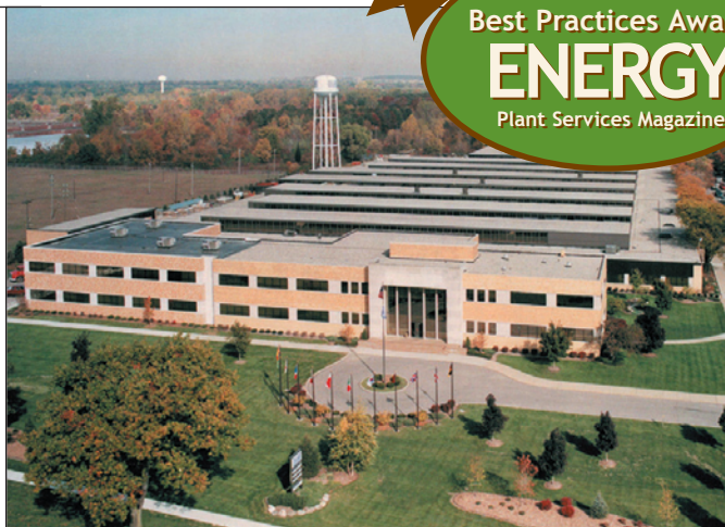
Durr Industries' 240,000-sq-ft North American headquarters and manufacturing plant replaced its 20-yr-old steam heating system with roof-mounted Cambridge Blow-Thru® Space Heaters.
